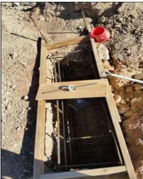
Winch Pad with Eyebolt Anchor and Rebar Cage
