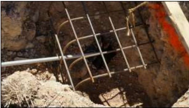
Hole with Anchor Rod and Cage
