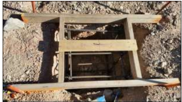
Base Plate Pad with Rebar
